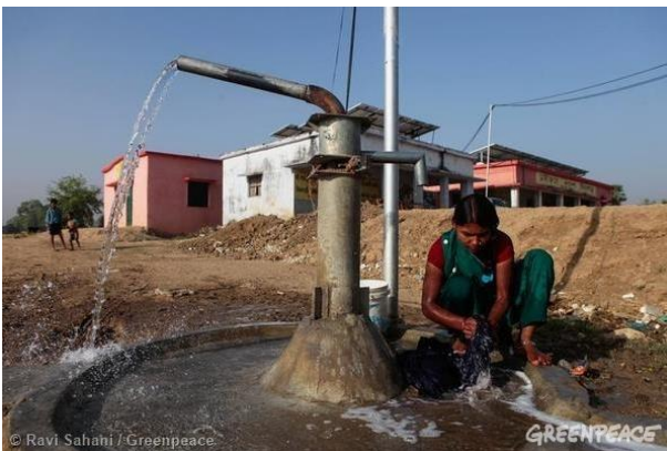
Fig.1 Solar DC pump in the first DC microgrid village of India.[19]
